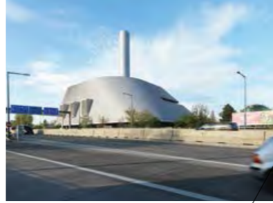
Fernheizwerk Arsenal, Arch. Markus Perenthaler, 2015, © Paul Ott
